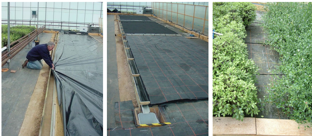
Photos 13 – 15. Laying polythene base layer (left), Experiment 2 plots with Florimat 2 and Mypex ‘Red Stripe’ (centre), and arrangement of three lines of T-tape offset up the slope with covered drain at the bottom (right).
