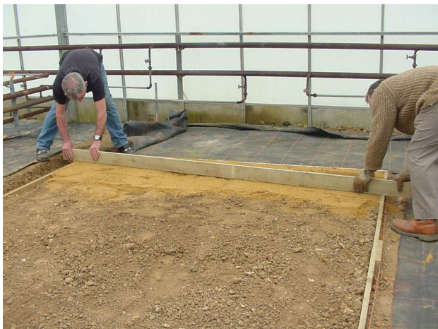
Photos 11 – 12. Filling and firming a smooth surface layer with sand.
