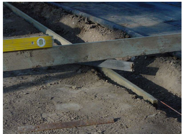
Photos 9 – 10. Construction of larger scale capillary flow beds. Creating 50 mm drop across the bed and a drainage channel.
