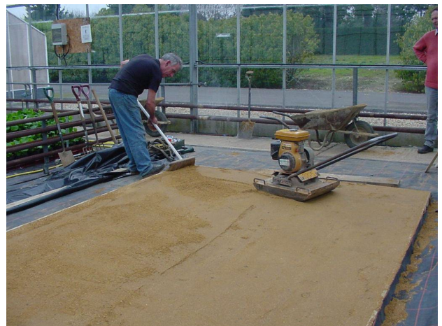
Photos 11 – 12. Filling and firming a smooth surface layer with sand.
